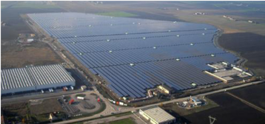
Fig. 1 – SunEdison's 70 megawatt (MW) photovoltaic (PV) power plant in Northeast Italy [3]
