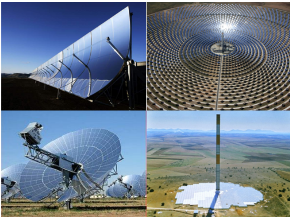
Fig. 2 – Solar Power concentration technologies
