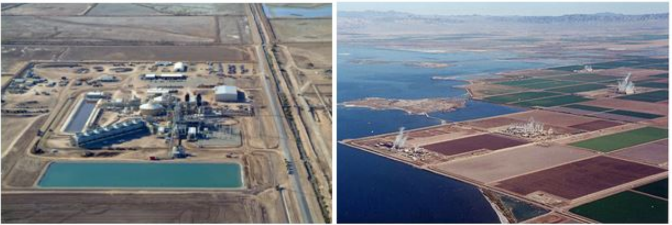
Fig. 5 – CalEnergy Generation’s Salton Sea Geothermal Plants, USA (from PowerTechnology)
