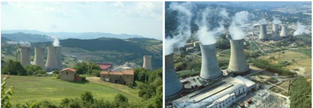
Fig. 2 – Larderello Plant in Italy (from EGP and ThinkGeoEnergy)
