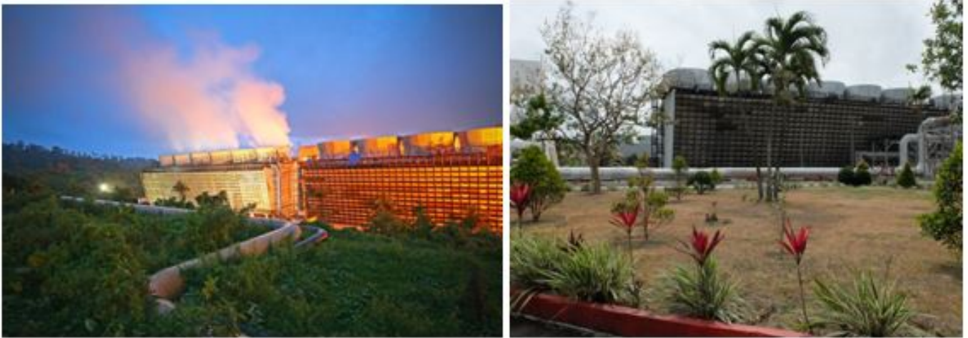
Fig. 4 – Makban geothermal power plant, Philippines (from: ThinkGeoEnergy)
