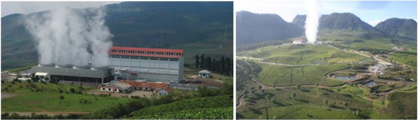
Fig. 10 – Wayang Windu Geothermal Power Plant, Indonesia
